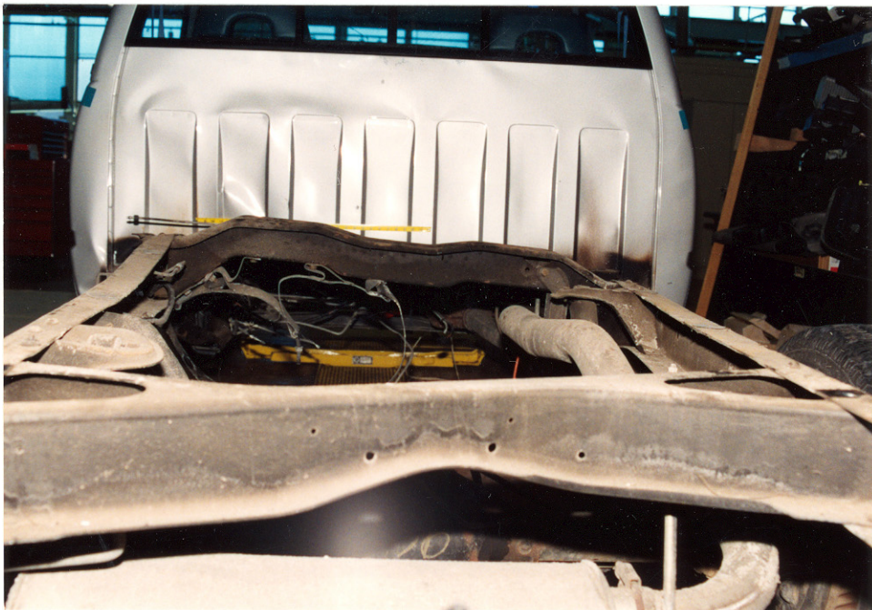
22. View of both frame rails and frame cross members illustrating the upward displacement from the CNG tank failure
